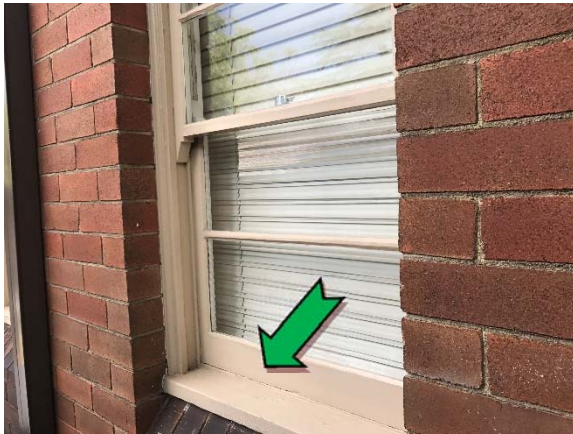
Photo 3. Interior, window frames, throughout –non asbestos-containing window caulking.
